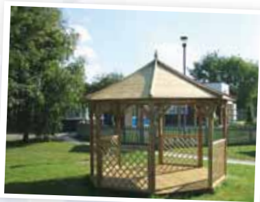
A winning design at Locking Primary School, Weston-Super-Mare, part funded by SCaRF and Friends of Locking Primary School
